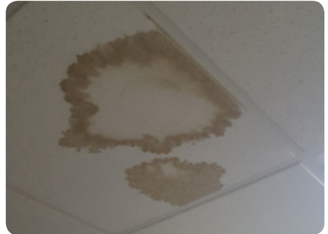
Water stains on ceiling tiles from condensate issues or roof leak.
