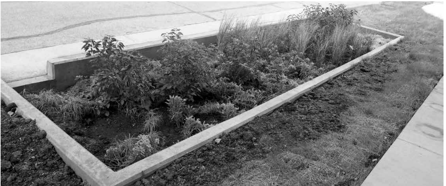
This street planter was recently installed at 73rd Avenue and Park View Boulevard to help filter storm water runoff before it gets to the Thompson Creek.
