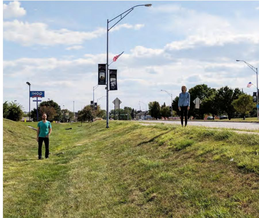
OPEN CHANNELS CONVEY STORMWATER AND ARE CONSIDERABLY LOWER THAN THE ROADWAY
