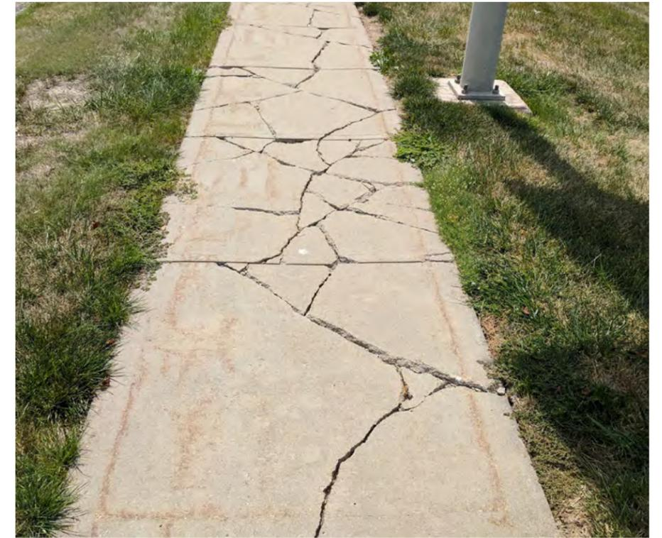
EXISTING 4' DETACHED SIDEWALK IN POOR CONDITION
