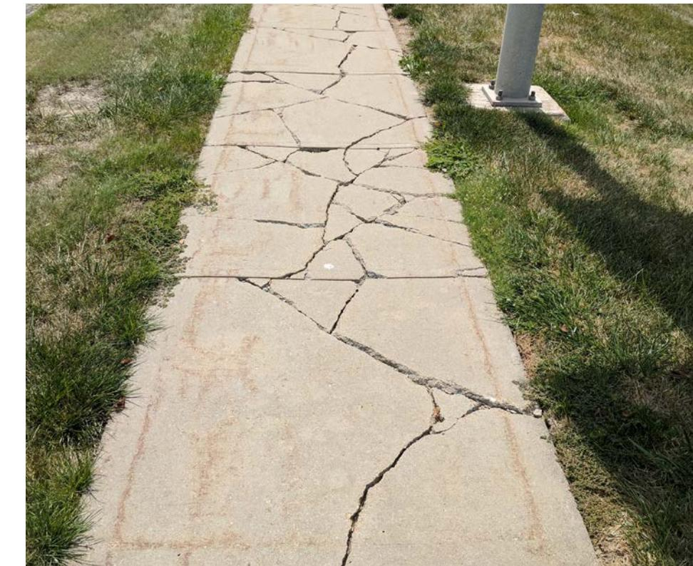
EXISTING 4' DETACHED SIDEWALK IN POOR CONDITION
