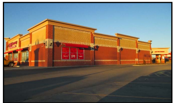
Multiple design elements and textures on all sides of the facility, including use of wall patterns, faux windows, elevation relief.
