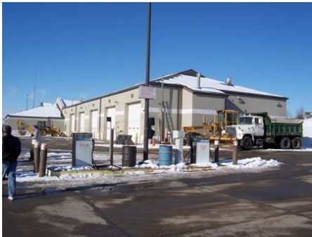
Fueling station and storage should have spill protection dike.
