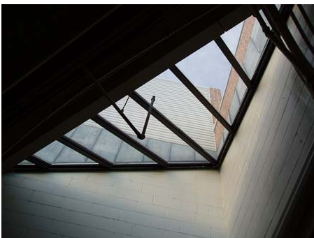
Skylights in apparatus room are prone to leaks.
