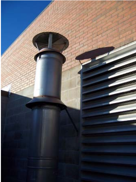
Boiler flue for the City Hall/Recreation Center should be extended so that it terminates two feet above the roof line.
