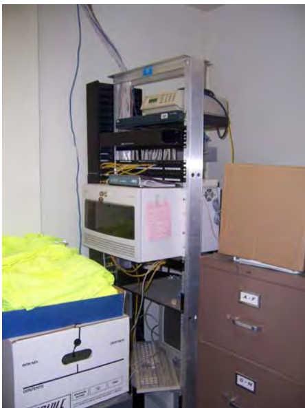
Server room is also used for storage, due to security issues access to the server should be restricted.
